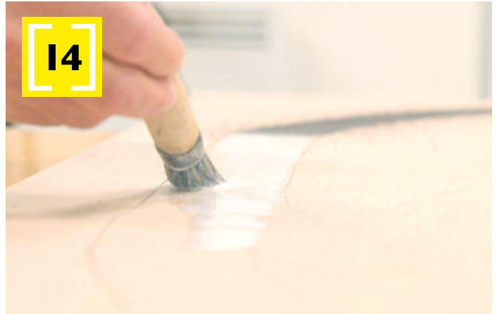
Using a 1" (300mm) paintbrush, apply the glue in between the lines you drew either side of the track. Do not worry if you go over the lines. Apply the glue in small sections, approximately 18" at a time.
